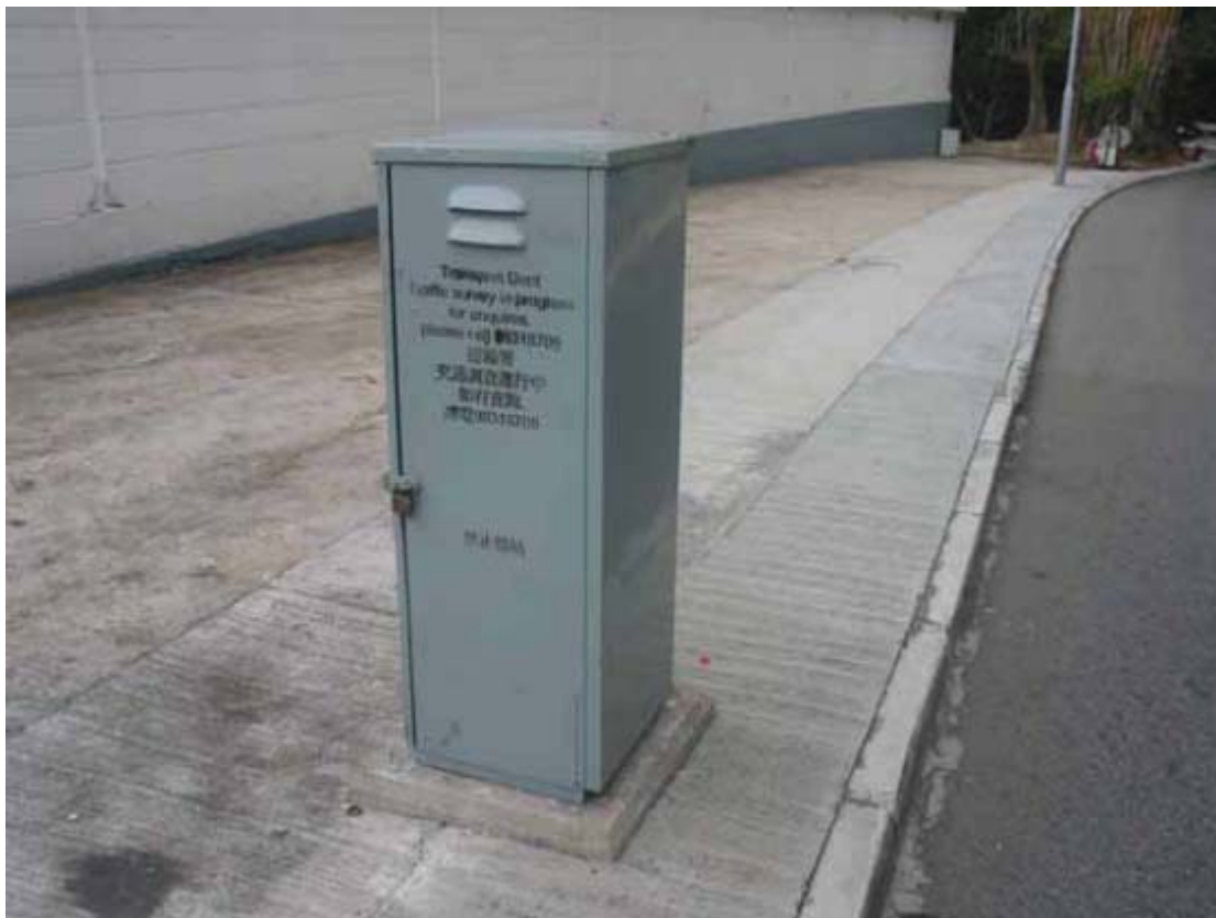
ATC Loop and Roadside Cabinet
