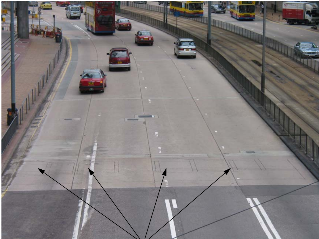
Loop Detector installed in concrete slab
